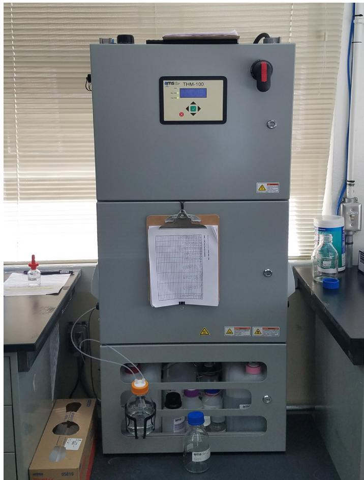
Online THM-100 analyzer installed at the onsite laboratory of the San Luis Obispo Water Treatment Plant.
