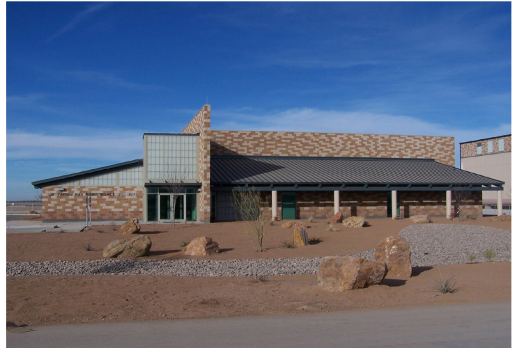
El Paso Water's Upper Valley Water Treatment Plant installed three automated online arsenic analyzers, which provide high-frequency, real-time data on arsenic contaminant levels in 30 minutes with sensitivity down to 1 ppb.
