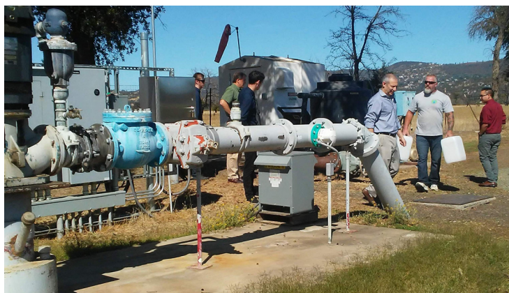
AMS pilot demonstration of its SafeGuard™ H2O Hexavalent Chromium [Cr (VI)] remediation system at California's Hidden Valley Lake Community Services District.
