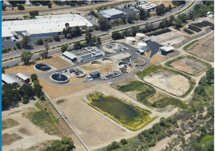
The City of Paso Robles operates a 4.9 mgd activated sludge wastewater treatment plant (WWTP) to meet the needs of 36,000 plus residents and a number of local vineyards and wineries. Treated wastewater from the facility is used for GWR to replenish the Paso Robles water basin and Salinas River. The facility faces stringent NPDES permit restrictions on effluent levels of total nitrogen (TN), microbiology and THMs.
